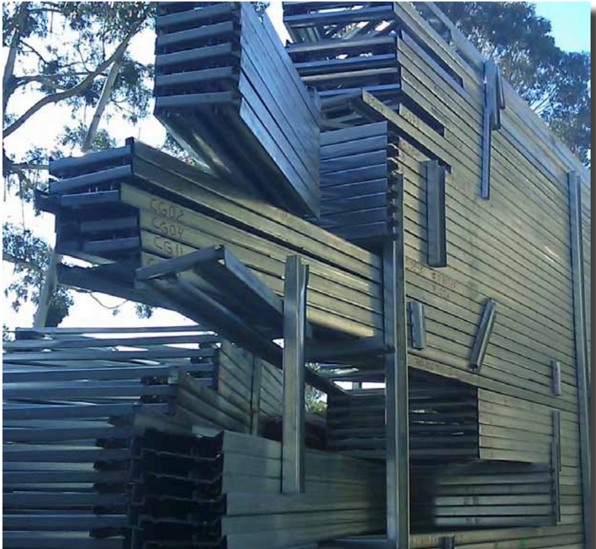
Above Image: Roof trusses delivered on-site.
