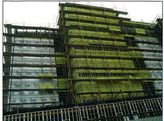
This Los Angeles, CA Crime Lab utilized the Team Panels system to accelerate production time and minimize on-site set-up errors.
